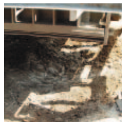
Von Roll blast floor panel AFTER explosion
